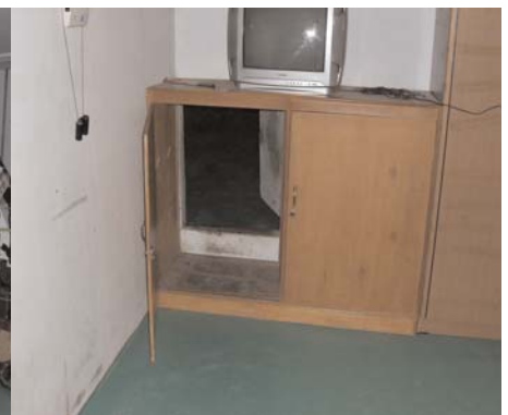
Hidden doorway to illegal plant
